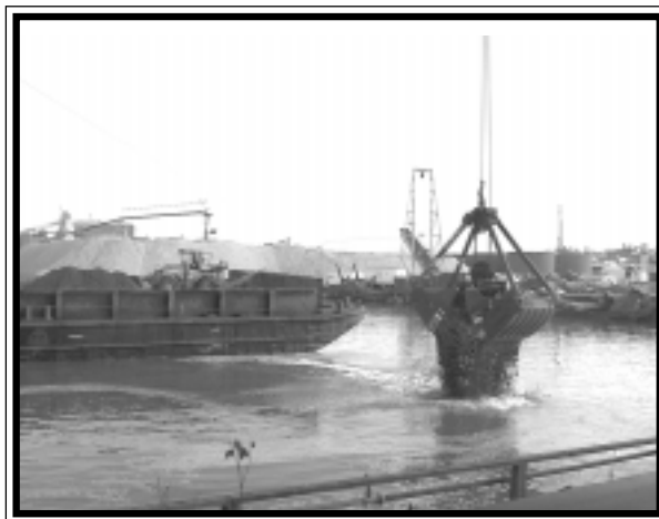
Capping material being placed on top of contaminated sediments at the Georgia Pacific Log Pond.
